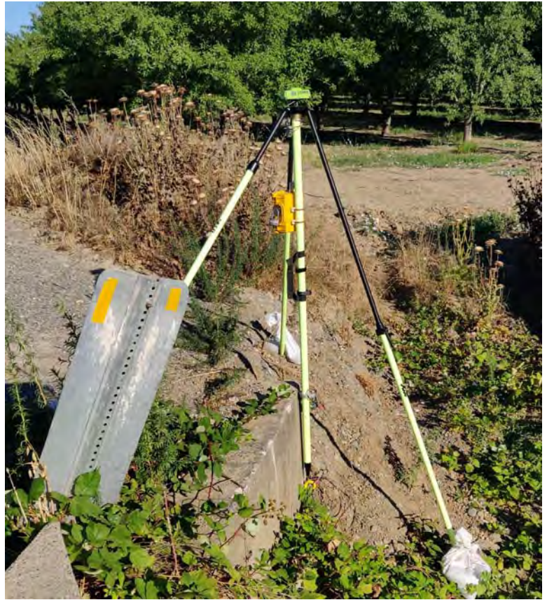
RTK base receiver at 5B35
